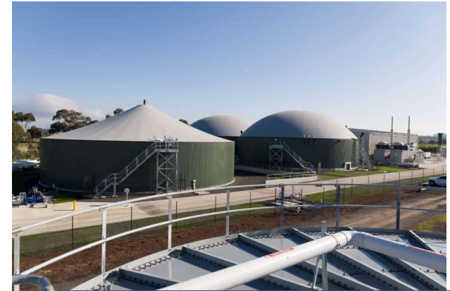
ReWaste Biogas plant Yarra Valley
