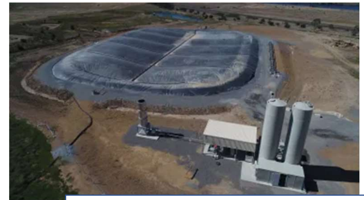
Southern Meats CAL, Goulburn, NSW
